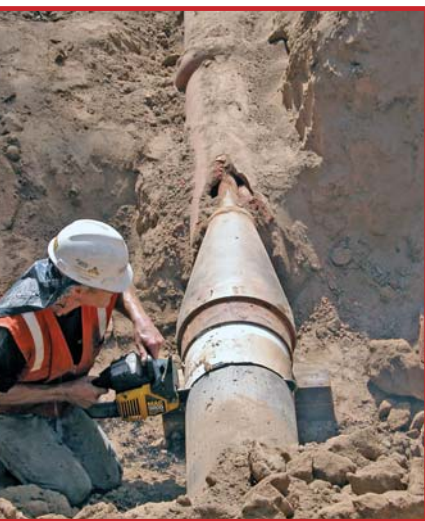
The bursting head is cut free
