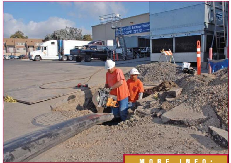
After the pull, a Nielson Construction crew cuts off excess pipe at entry pit.
