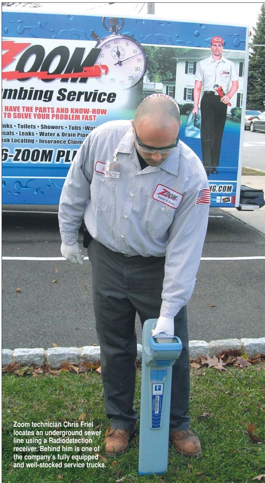
Zoom technician Chris Friel locates an underground sewer line using a Radiodetection receiver. Behind him is one of the company's fully equipped and well-stocked service trucks.
