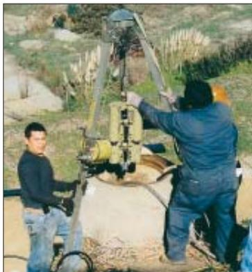
**Technicians with The Lighthart Corp. set up at one of the manholes along the route from the Loyola Marymount campus to the main city sewer.**
