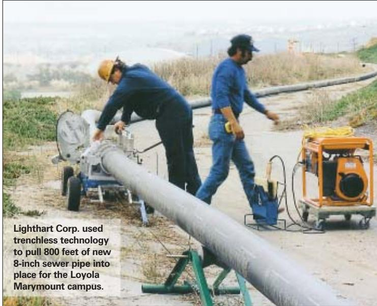
**Lighthart Corp. used trenchless technology to pull 800 feet of new 8-inch sewer pipe into place for the Loyola Marymount campus.**
