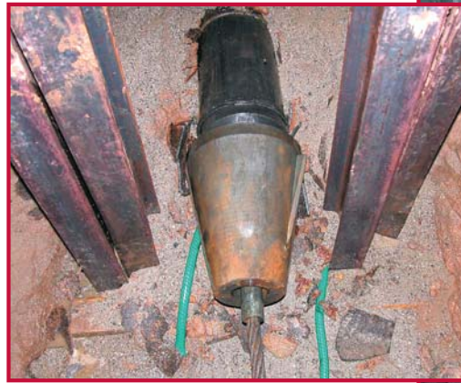
This pulling assembly was used to burst the old pipe.
