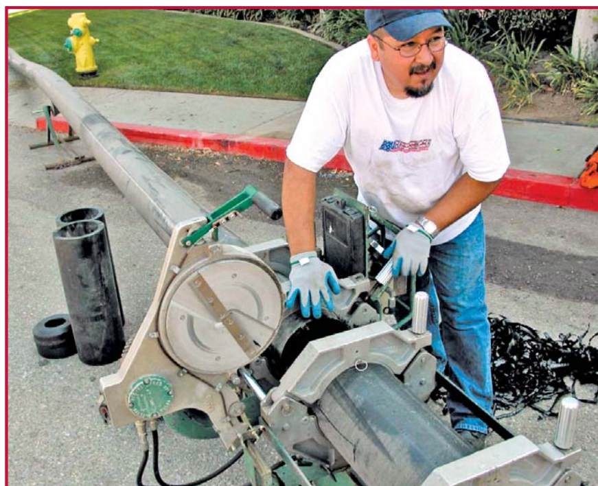
A technician fuses sections of 8-inch SDR17 HDPE pipe.
