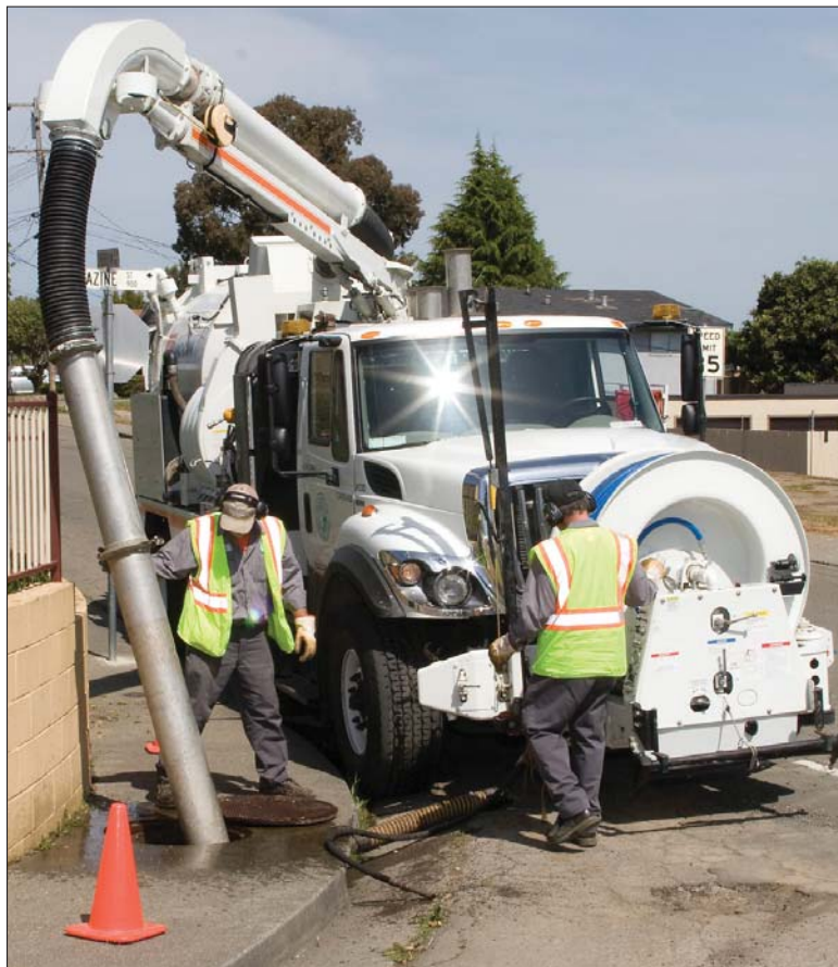
Collection systems technician Scott Ransford prepares a Model 1065 cable machine from Spartan Tool to cut a root located by a camera crew.
