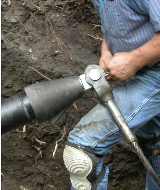
Figure 6 Clevis & pulling-eye head connection
