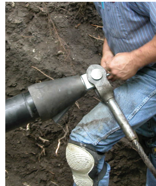
Figure 6 Clevis & pulling-eye head connection
