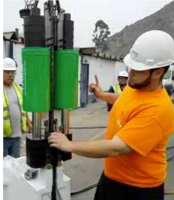
Figure 6 Pulling cable slack to help insert cable to lower grippers
