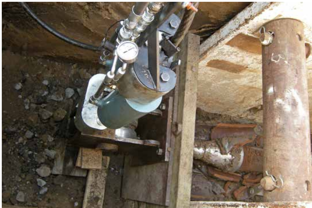
Figure 9 M100 with trench box
