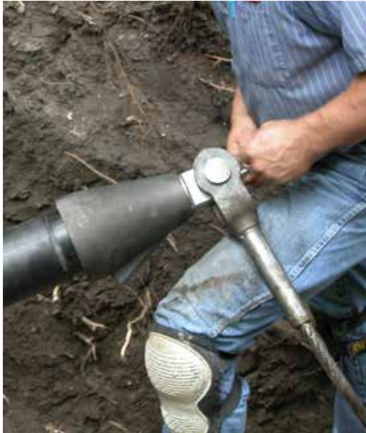
Figure 6 Clevis & pulling-eye head connection
