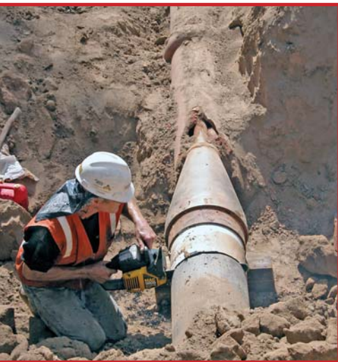
The bursting head is cut free
