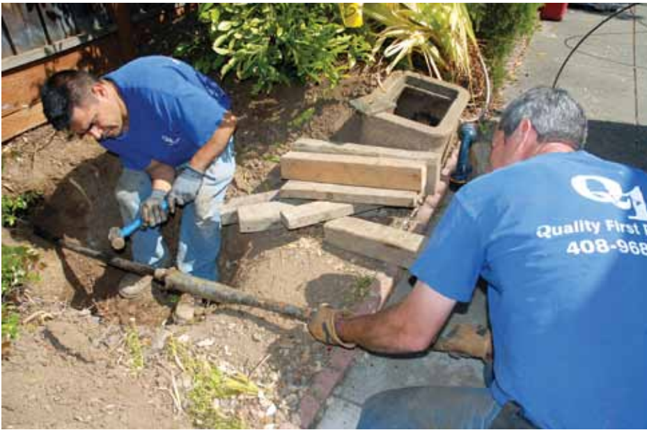
LEFT: Atanacio Francisco hammers the last length of galvanized pipe off the bursting head as Bob Zamaroni hangs on and pulls. The stop plate is on top of the utility box. RIGHT: Pull completed. A 2-inch-long Acme screw adaptor attaches the 1-inch HPDE pipe behind the 16-inch-long bursting head with 6-inch-long slitting blade welded at rear. Note the 2-degree bend in the cable at the swage and the length of the swage before it reaches the inverted slitting blade.
