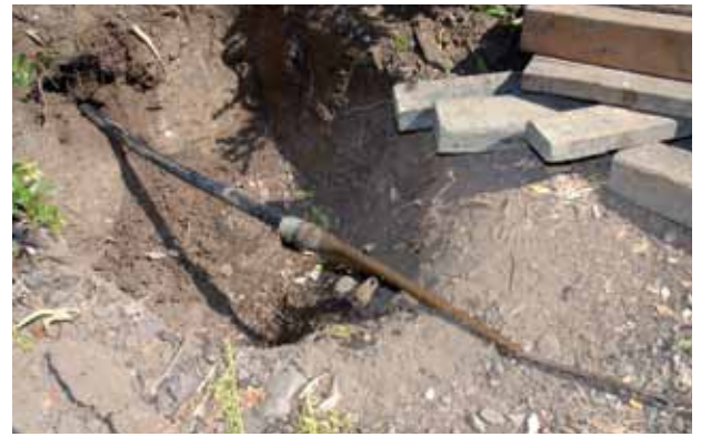
LEFT: Atanacio Francisco hammers the last length of galvanized pipe off the bursting head as Bob Zamaroni hangs on and pulls. The stop plate is on top of the utility box. RIGHT: Pull completed. A 2-inch-long Acme screw adaptor attaches the 1-inch HPDE pipe behind the 16-inch-long bursting head with 6-inch-long slitting blade welded at rear. Note the 2-degree bend in the cable at the swage and the length of the swage before it reaches the inverted slitting blade.
