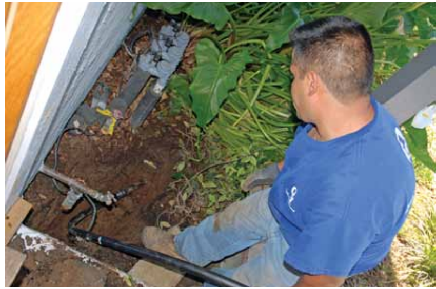
Technician Atanacio Francisco from Quality First Plumbing helps guide the 1-inch HDPE replacement pipe into the pit at the start of the pull. The ACME coupling attaching the pipe to the rear of the bursting head is visible just past the spigot. (Photos courtesy of TRIC Tools)
