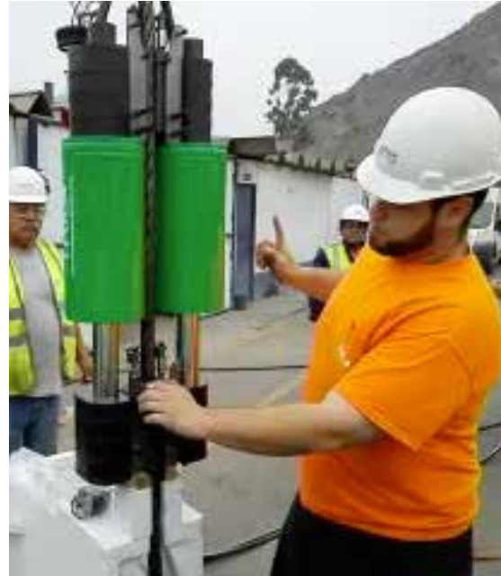
Figure 5 Pulling cable slack to help insert cable to lower grippers
