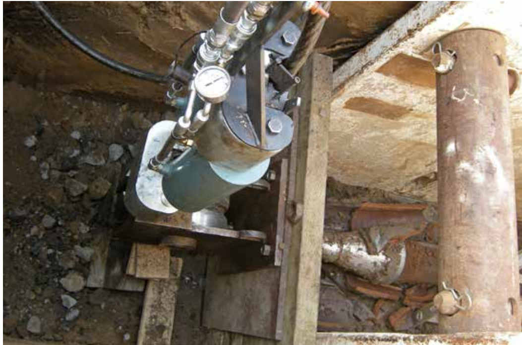
Figure 8 M100 with trench box
